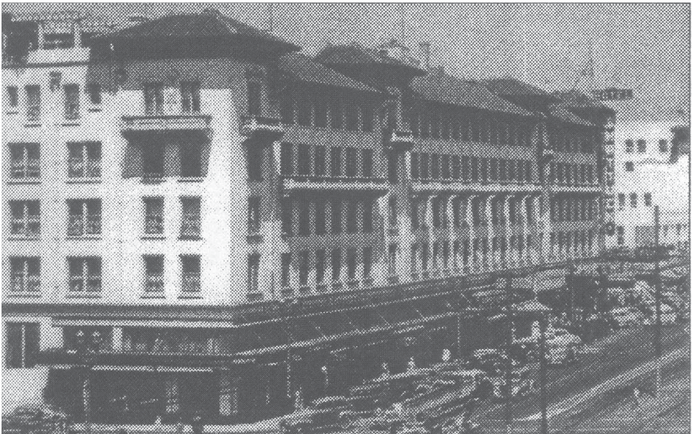
Figure 15: This historic photo of the Shattuck Hotel illustrates several principles of façade design. The articulated roof profile and façade planes and the Hink's canopy lend interest and a "human" scale to what is in fact a very large building (Source: Berkeley Architectural Heritage Association).
