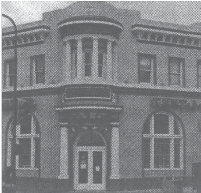
Figure 50: On corner sites, the corner should be emphasized as a focal point. This building combines a chamfered corner with a more elaborate architectural treatment.
