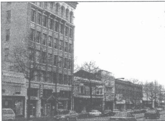
Figure 54: Historic structures on University Ave.
