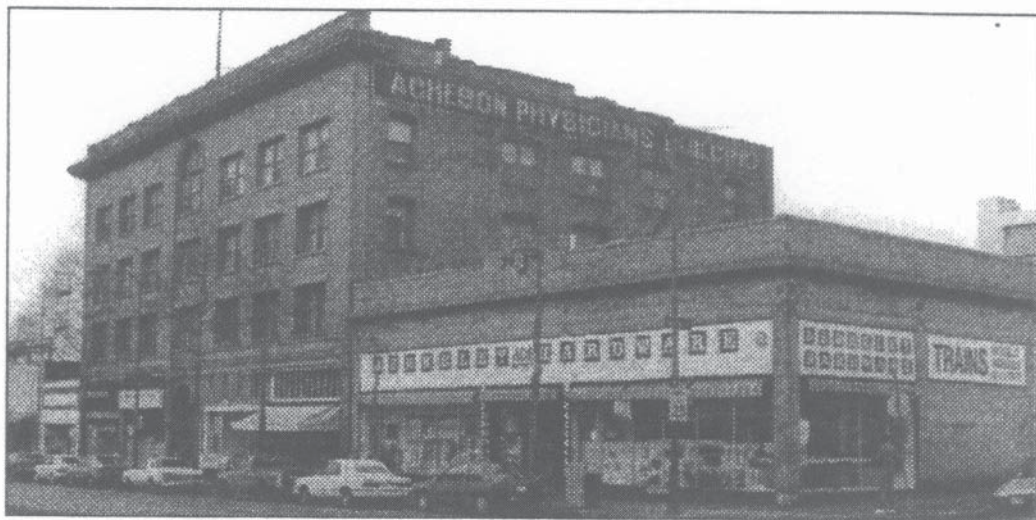
Figure 56: Historic structures on University Ave.
