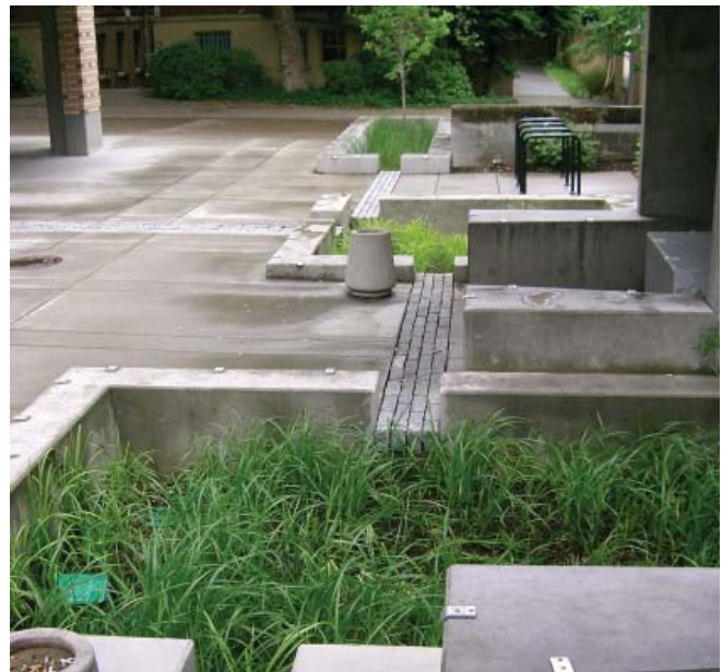
Figure 47: “Rain Gardens”. On-site rainwater retention features can be attractive landscape elements, such as the “rain garden” shown. Rain gardens hold most water below landscaping or rockery but can also fill with a few inches of visible water above during heavy rains.
